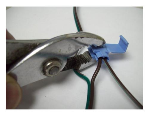
Use pliers to push the metal spade down until it is flush with plastic. This is what makes the electrical connection between the two wires.
